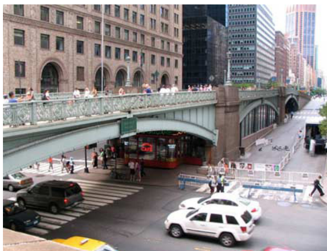
Park Avenue Viaduct (1919) Manhattan, Nova Iorque, EUA Warren & Wetmore; Reed & Stem
