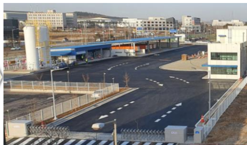
Tube Trailer Filling Station
